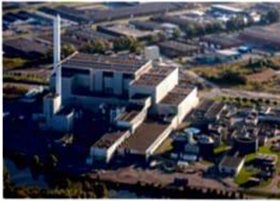
A recycling and waste-to-energy plant for waste that is not exported
